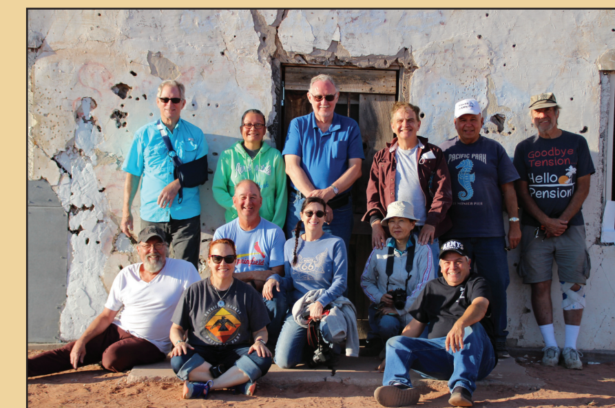
This group journeyed to the trading post in September 2020 to begin stucco repair and complete other chores.
